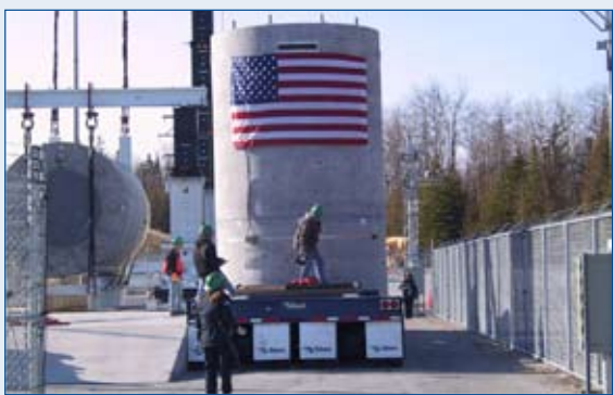
Workers move a cask loaded with spent nuclear fuel from the shut-down Big Rock Point nuclear plant to a temporary onsite storage facility. The waste will remain at the Michigan site until the federal government develops a facility for storing or disposing of the nation's spent fuel. Photo credit: Entergy Nuclear.
